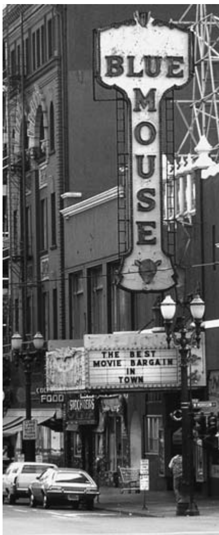
Figure 1.11. Blue Mouse theater, Portland, Oregon, with original 1912 signboard, immediately prior to demolition, 1977.
